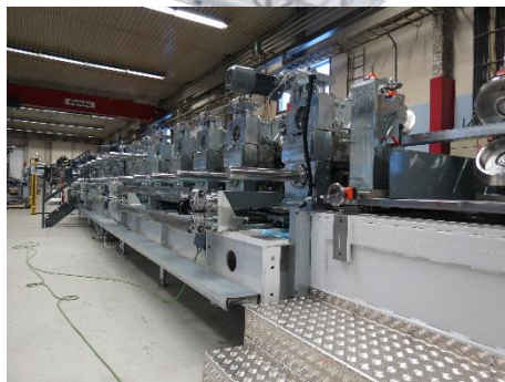
UNIT CONTROL (PLC) Machine functions: machine I/O, motors, valves, sensors etc.
